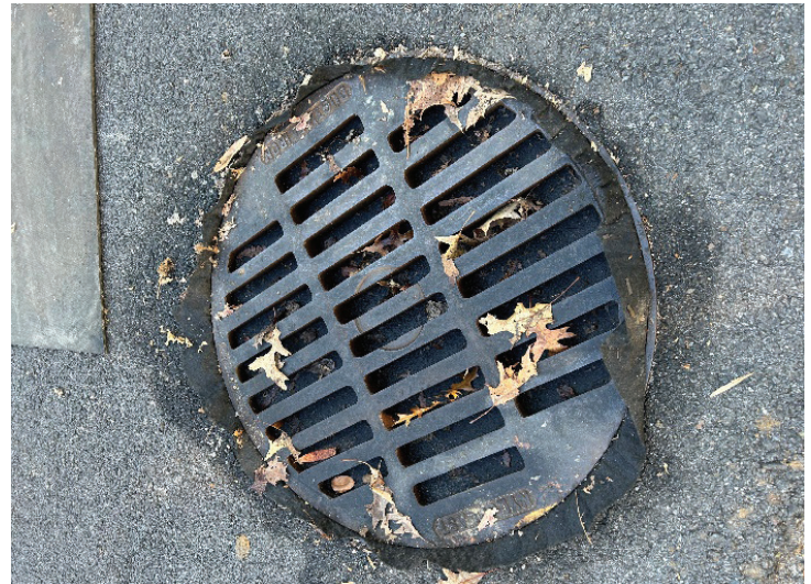
A storm drain with mesh underneath for catching resin and other materials.
