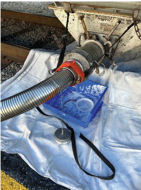
A catch pan with a tarp underneath to prevent spills during loading/unloading.
